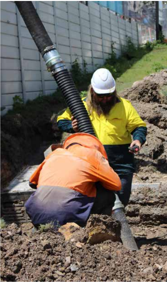
Vacuum Excavation operators under-taking service locating operations to assist local developers in avoiding striking underground utilities as they work!
